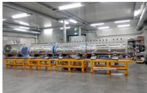
DTL assembled on site
