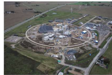
Fig. 2: Photo of the ESS site.
