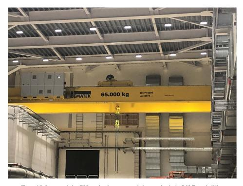
Figure 6.3: Largest existing ESS overhead crane currently in operation in the D02 Target building
